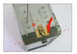
Apply the springs (D) to the 5. 2-DIN Navigation using the mounting hardware (D) as neccessary
